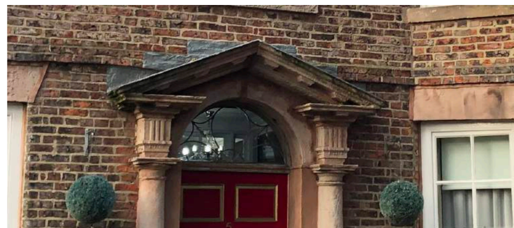
TUSCAN DOOR CASE AND PORTICO, FANLIGHT AND LANTERN, VIEW FROM WESTOE VILLAGE
